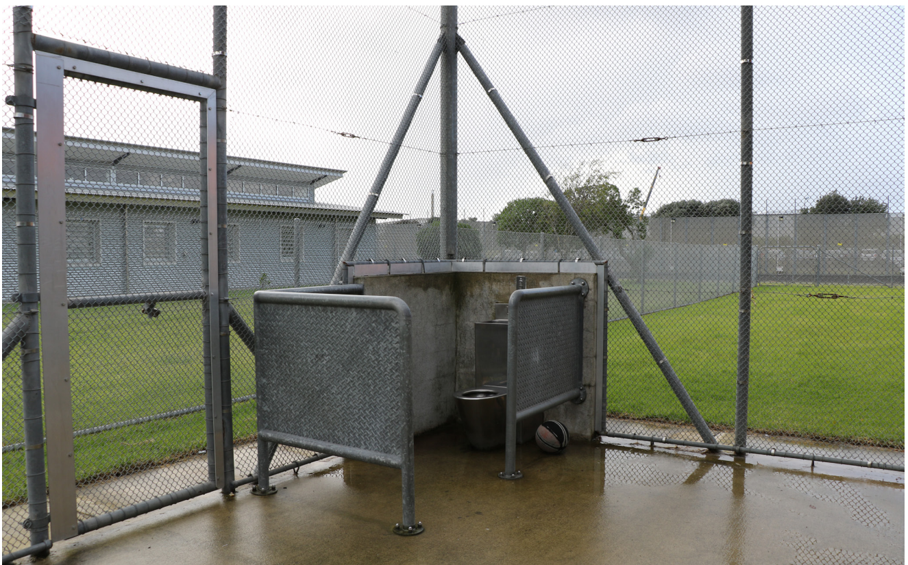
A toilet in an outdoor exercise yard.
